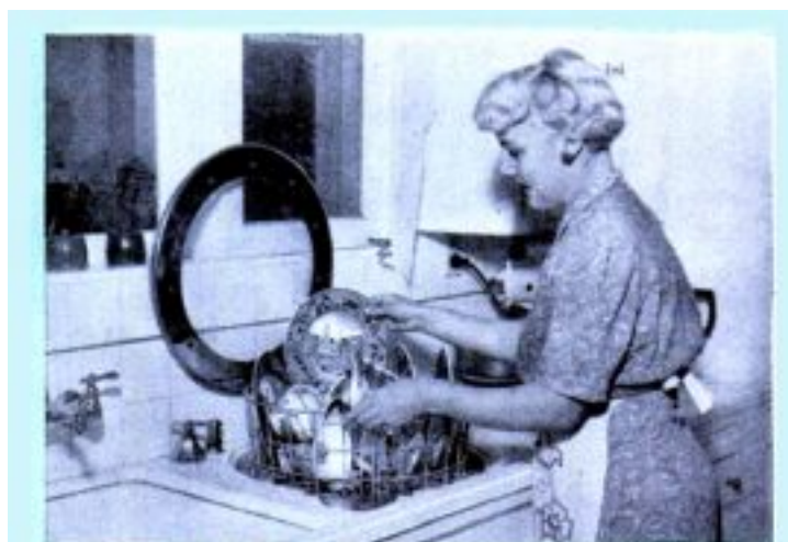
AUTOMATIC DISHWASHING is done in a new sink accessory without a motor, belts, or a whirling spray arm, operation being simply on city water pressure. The machine is a product of Q. E. D. Dishwasher Co., of Alhambra, Calif.
